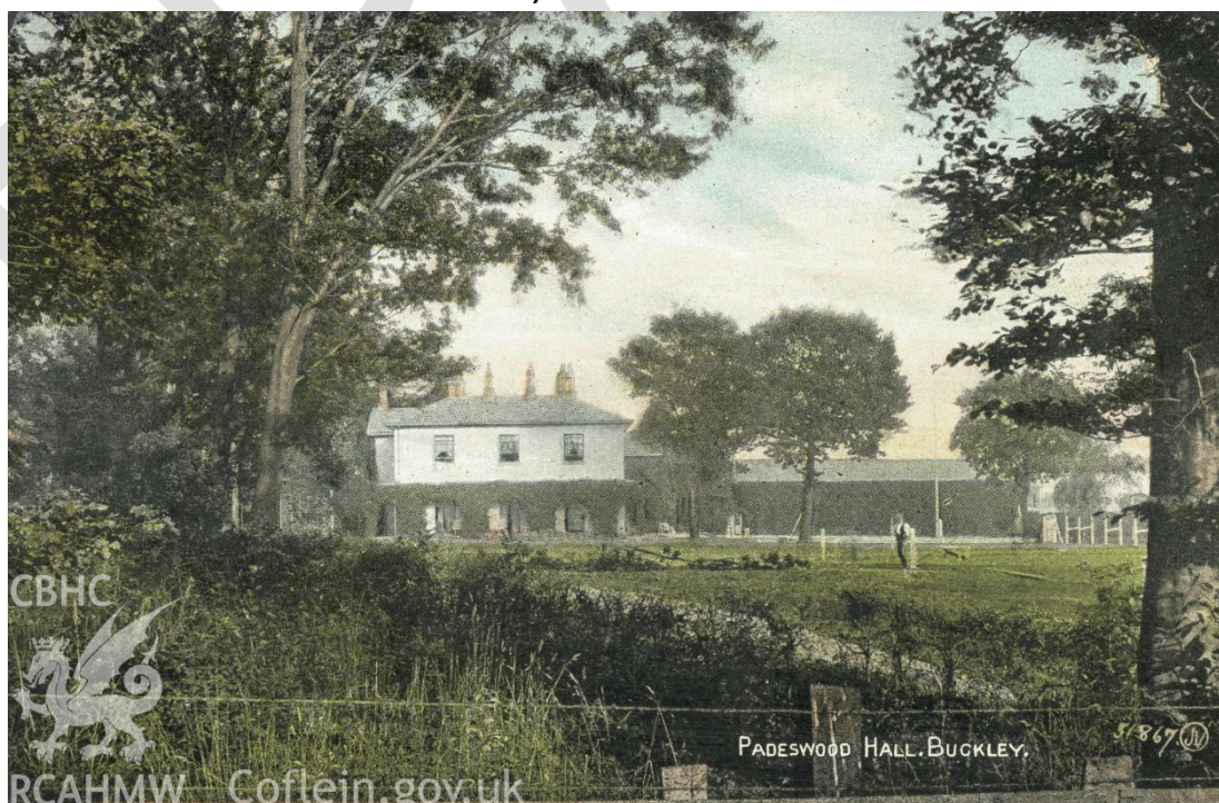
Figure 2 1905 Postcard of Padeswood Hall (Royal Commission on the Ancient and Historic Monuments of Wales)
