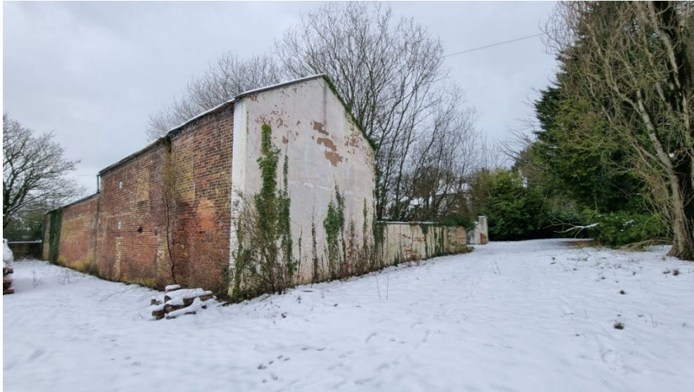
Figure 5 Padeswood Hall Farm Buildings, view to south west
